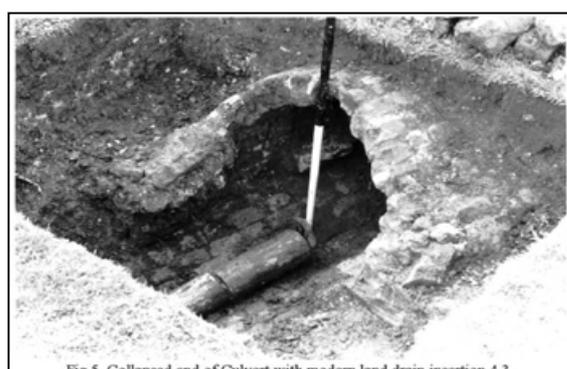
Fig. 5. Collapsed end of Culvert with modern land drain insertion 4.3.
